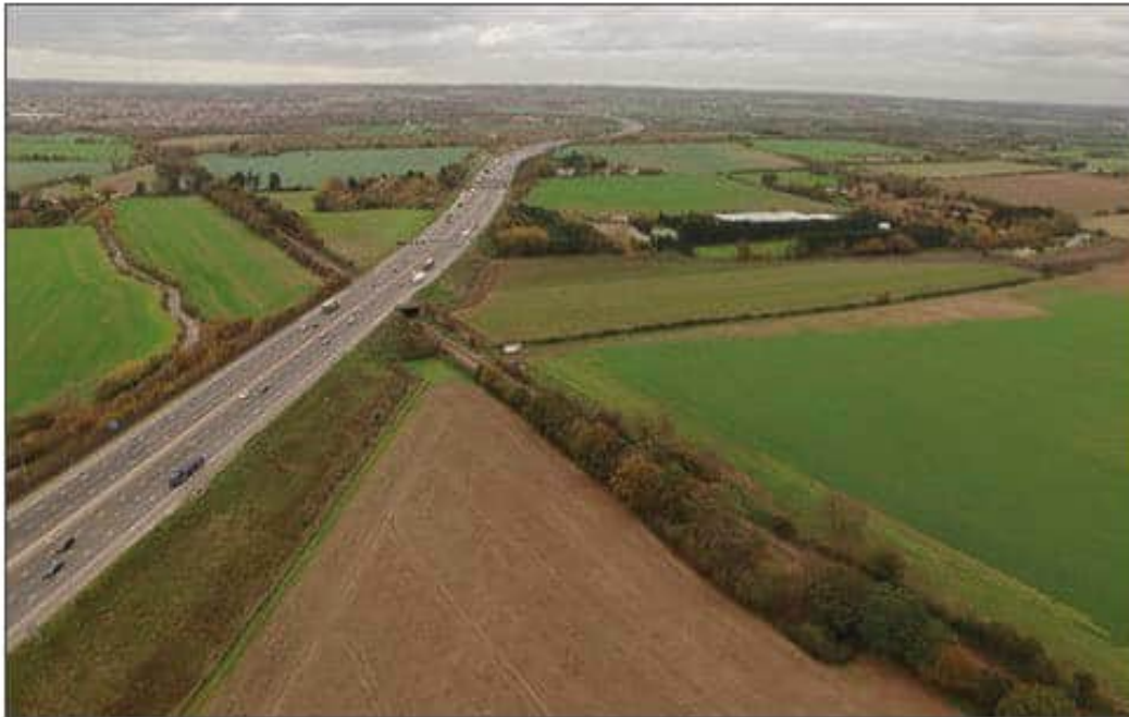
Figure 5-34. Existing M25 junction looking north
