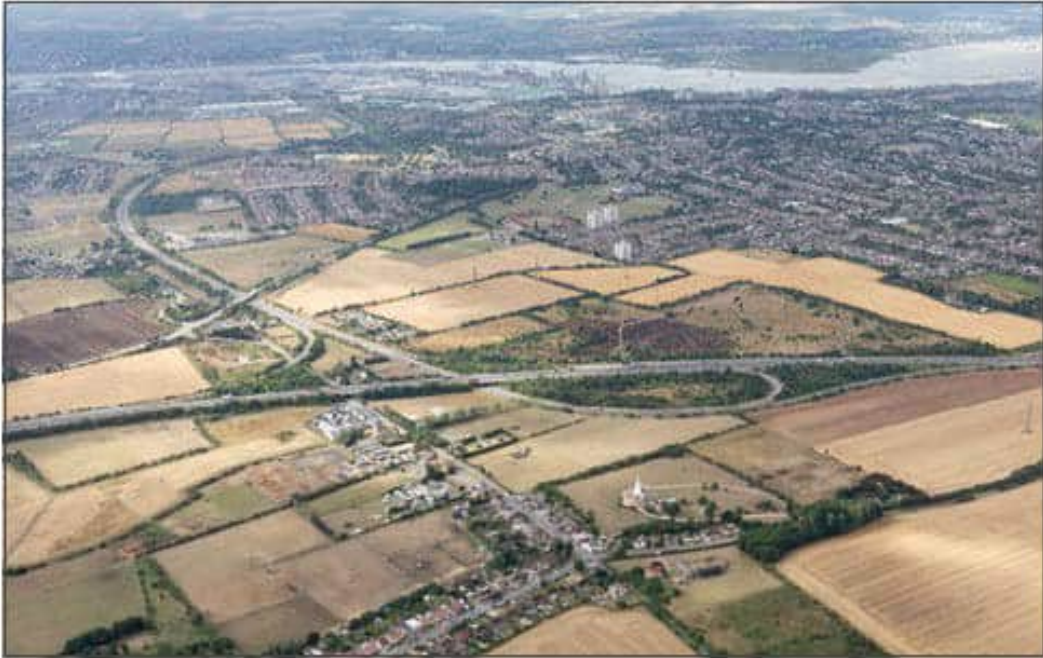
Figure 5 23. Existing A13 junction, looking south
