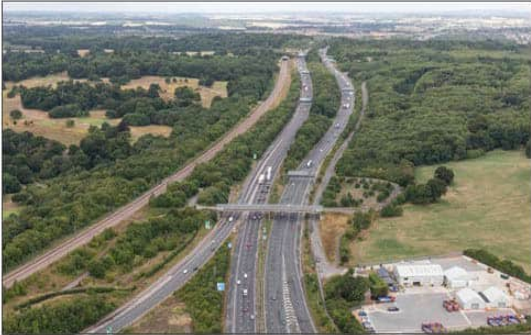
Figure 5 7. Existing M2/A2 along the A2 near Park Pale bridge, looking west
