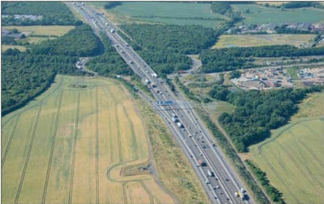
Figure 5 38. Existing view of M25 between junction 29 and 30, looking north
