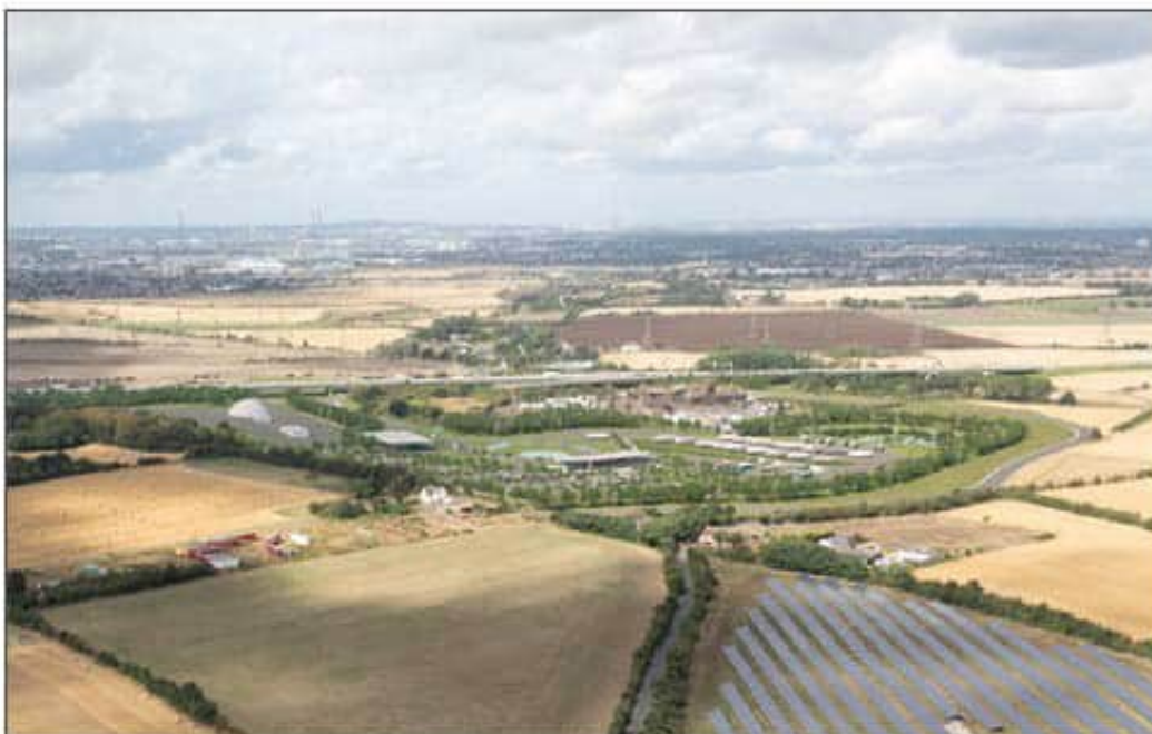
Figure 5 21. Proposed Tilbury junction and a proposed rest and service area, looking west
